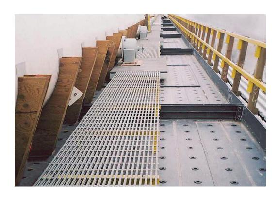
Midwest Plank™ hot water basin panel system interlocks and overlaps to form a safe, strong working surface on your cooling tower. Manufactured of pultruded fiberglass reinforced polyester, the lightweight, high strength and corrosion-resistant design offers quick, easy installation.
