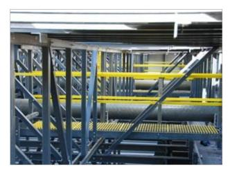
Midwest Cooling Towers offers fiberglass equipment access walkways and work platforms for permanent or temporary use. They are corrosion-resistant, slipresistant, ultraviolet-resistant, strong, lightweight, and fire-retardant.
