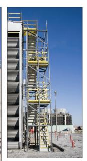
The Midwest pre-engineered fiberglass stairway provides safe, easy access to your cooling tower. Its lightweight, yet rugged design offers quick, easy installation.
