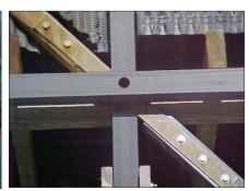
Midwest Cooling Towers pultruded fiberglass structural shapes allow you to replace deteriorated wood columns, beams, and decks on your cooling towers with strong, lightweight, rot-resistant fiberglass.
